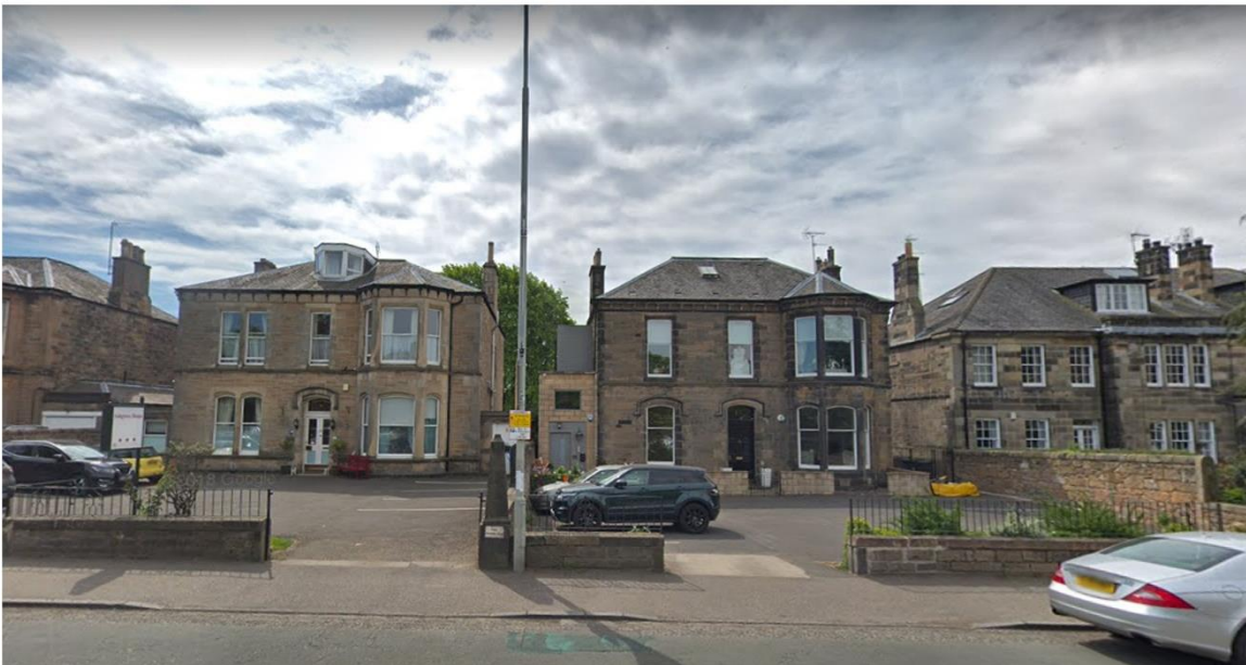
Figure 4.3 – The above shows the front elevation of 13 Osborne Terrace.
